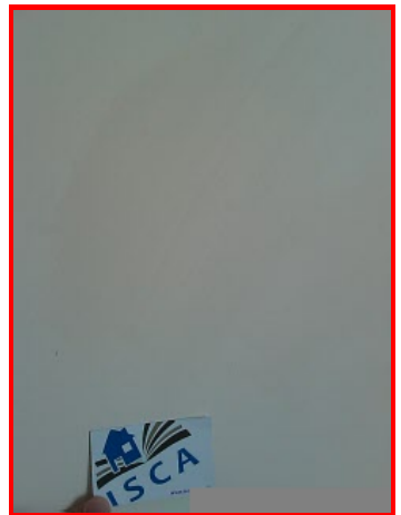
Bedroom 1 Walls Wall finish - Paint touched up (opposite bed)
