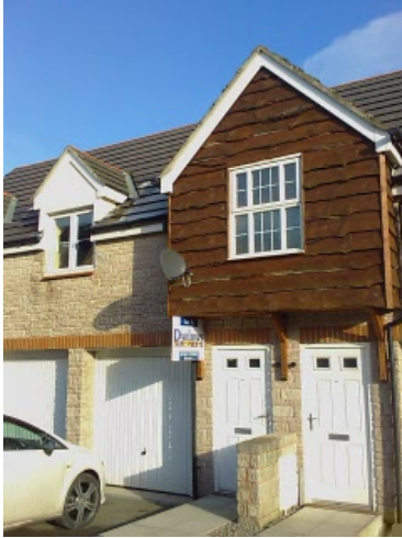
Front of building
