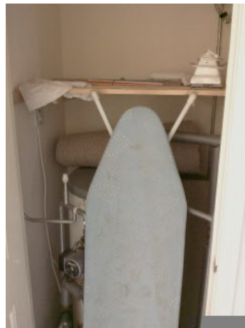
Airing cupboard, Ironing board
